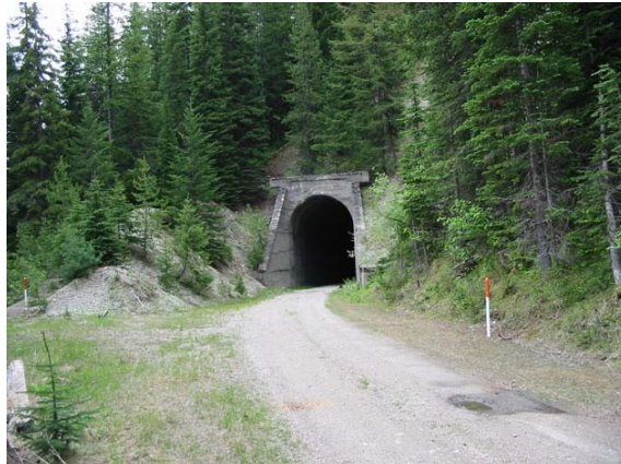
Northern Pacific Tunnel 1 (Borax)
