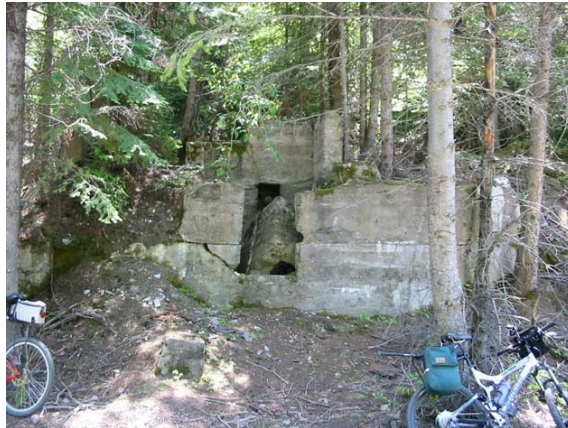
Dorsey Water Tower Remnants
